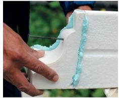
14. If necessary, fix the elements between by means of neatly screwed screw.
