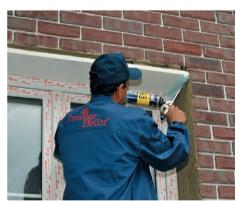
7. At the place where the elements meet each other, apply adhesive foam to the entire depth of the seam. The thickness of the glue-foam seam should be 1.5-2.0 mm. Remains of adhesive foam should protrude from the seam by 2-3 mm.
