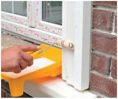
18. Mounted decorative elements are required to substantiate using primer, recommended by the manufacturer for further decorative finishing.
