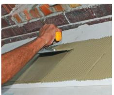
3. Materials and products for fastening decorative parts to the building base must ensure a rigid connection between themselves (without gaps). In all cases, glue is a mandatory component of fastening.
