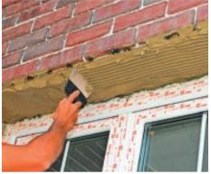
2. Prepare the slope element for installation. Apply an adhesive construction mixture to the places where decorative elements are installed.
