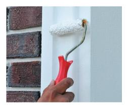
19. After completing the installation of the elements decorative finishing of a facade is done (using acrylic paints or decoration, using decorative facade plasters).
