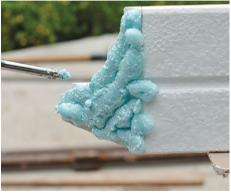
12. Layer of glue-foam with a diameter of 10 mm should be applied to the entire surface joint of the element.
