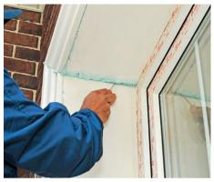
13. After complete drying, it is necessary to cut off the excess adhesive foam (2 mm), freeing the surface for applying the restoration mixture
