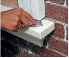
16. Cover the prepared joints by restorative mixture "DarMix" by spatula to a depth of 2-2.5 mm.
