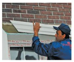
11. Apply the adhesive mixture to the place of installation of the decorative element.
