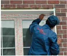
Check with a square the correctness of the angle slope in relation to the plane of the window.
