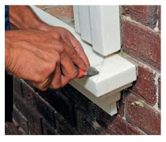
15. Free all connecting seams of 2 mm in width and depth from adhesive foam, for subsequent application of "DarMix" restorative mixture.
