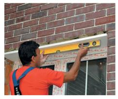
5. Check horizontality of the glued decorative element with a construction level.
