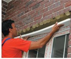
4. The architectural detail, with freshly applied adhesive mass, is manually pressed to the construction base. The pressure continues until the entire adhesive mass has reliable contact with the base.
